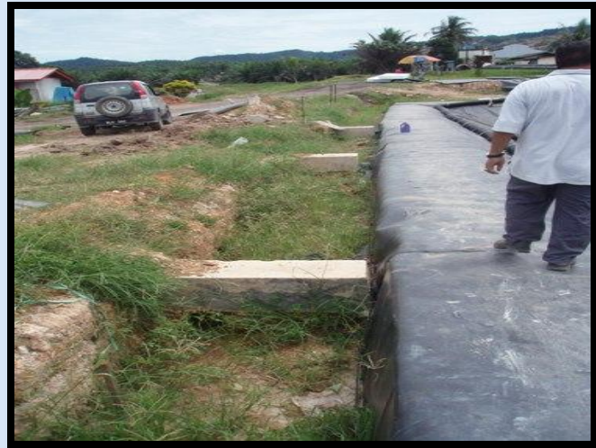
Anchor trench near to effluent pipes.
