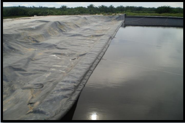
Deployment of the 1.5mm thk. HDPE Cover
